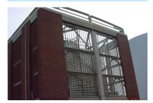
The Chiller Plant at the University of North Carolina is protected with a coating system that includes Series 1070 Fluoronar which offers superior color and gloss retention.
