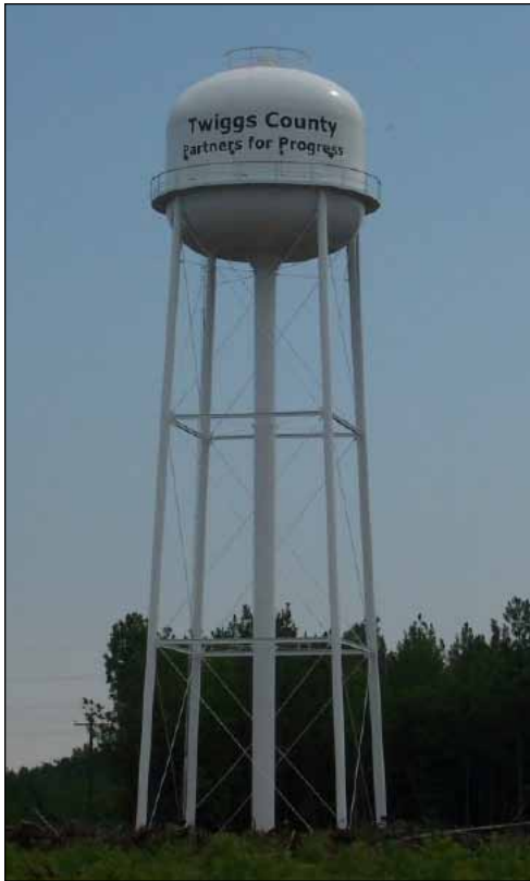
Series 700 HydroFlon, a fluoropolymer polyurethane finish coat, protects the exterior of the Twiggs County water tank in Georgia from UV light degradation, abrasion and chalking.
