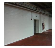
After photos of the walls at the Smithfield Foods plant in Landover, MD. Now protected with a Stranlok fiberglass-reinforced coating system, the walls can withstand thermal shock from daily high-pressure steam cleaning.
