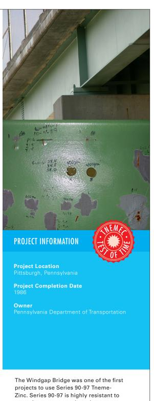
projects to use Series 90-97 Tneme-Zinc. Series 90-97 is highly resistant to corrosion, easy to apply and can cure at lower temperatures. It has kept the Windgap Bridge looking great for more than 30 years.
