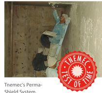
Shield System, including the trowel application of Series 434 Perma-Shield H<sub>2</sub>S at 1/8" to the concrete substrate (bottom photo), protects the Robinson Street Lift Station
