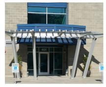
Series 1077 Enduralume, an acrylic polyurethane with a metallic finish, protects the exposed structural steel at the Port of Seattle Terminal 46 in Washington state.
