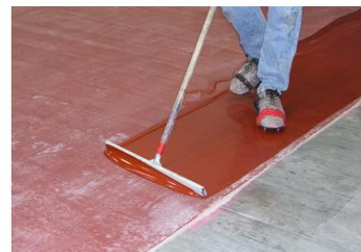
Engineers for PepsiCo.'s Gatorade bottling plant expansion project in Tolleson, AZ chose Ultra-Tread, a polyurethane modified concrete floor topping, to provide thermal shock resistance for approximately 45,000 square feet of poured concrete floor surfaces in the bottling facility.
