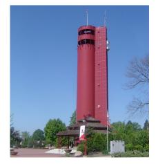
Series 700 HydroFlon, a fluoropolymer polyurethane finish with excellent color and gloss retention, protects the exterior of the standpipe in Peoria Heights, IL.
