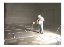
Series FC22 Epoxoline was used to coat the interior of the Palmer 500,000 Gallon Tank in Missouri City, TX because of its rapid cure capability and high-build substrate protection.
