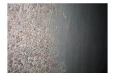
Because areas of the Oneota Street Pump Station in Duluth, MN were severly deteriorated, Series 218 MortarClad was used to resurface and repair the concrete.
