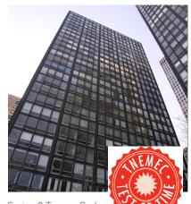
Series 6 Tneme-Cryl, a water-based acrylic emulsion in a charcoal black color, protects the entire exterior steel curtain wall of the towers at 860-880 Lake Shore Drive in Chicago, IL.
