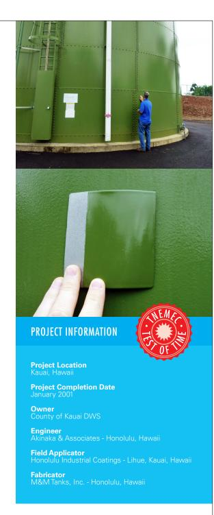
After almost 20 years of exterior weathering in tropical sunlight, hot weather, humidity and frequent rains, the gloss and color of the Series 700 HydroFlon topcoat applied to the Kakela water storage tank in Kauai, Hawaii, remain intact with no noticeable change. Photos shown were taken in 2011.
