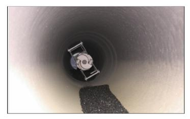
The compressed air used for blasting shall be free of water and oil. Adequate moisture traps and separators should be used to ensure elimination of all contaminants. Cleanliness of the air supply should be checked daily by operating the line without abrasive media through blotter paper for 30 seconds (reference ASTM D 4285). If oil or water appears on the cloth, the traps and separators should be cleaned until subsequent tests prove satisfactory.
